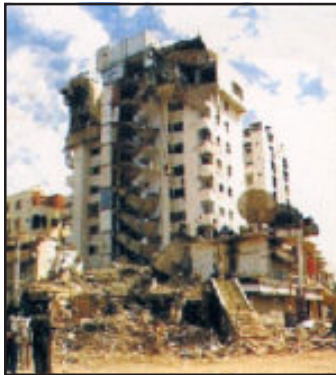
Fig. 3.3a: Destruction caused by an Earthquake in Gujarat
